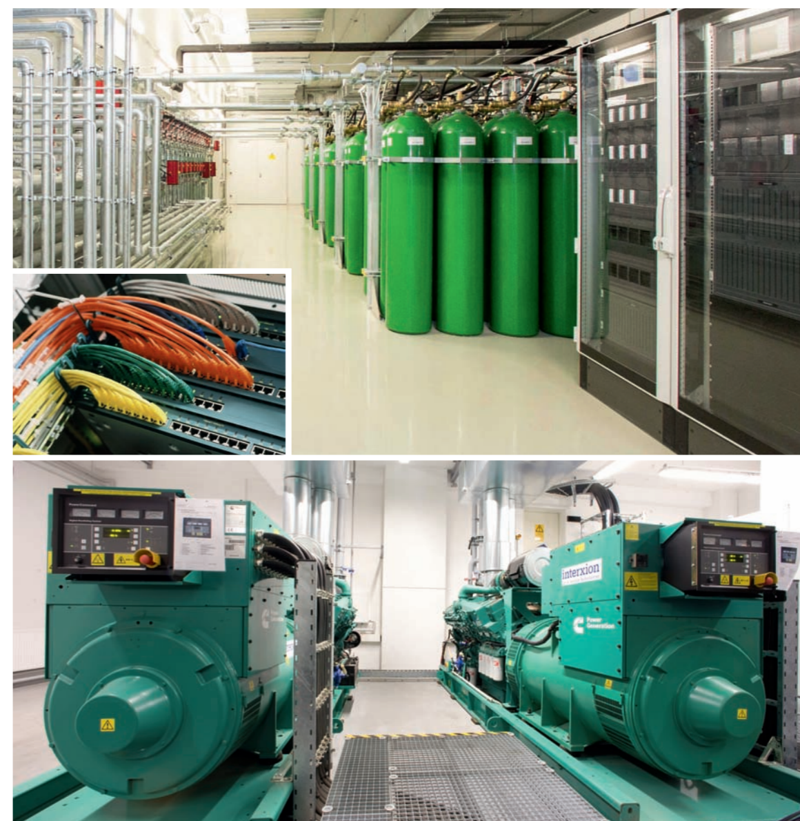
Interxion relies on state of the art safety-engineering, e.g. extinguishing gas systems (picture above) and redundant backup generators for interruption-free continuous operations (picture below). The Frankfurt campus offers direct connections to over 450 carriers and internet service providers (small picture). Picture on the left: State-of-the-art Interxion campus in Frankfurt.
